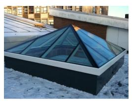
As part of a large project the team at Cambs Glass supplied and installed this modern thermally isolated pyramid rooflight to a flat roof extension of a school refractory. The rooflight was designed by our in-house team to be stick built on site thus minimising the panel and bar size and allowing easy transportation to site from our location in Suffolk.
